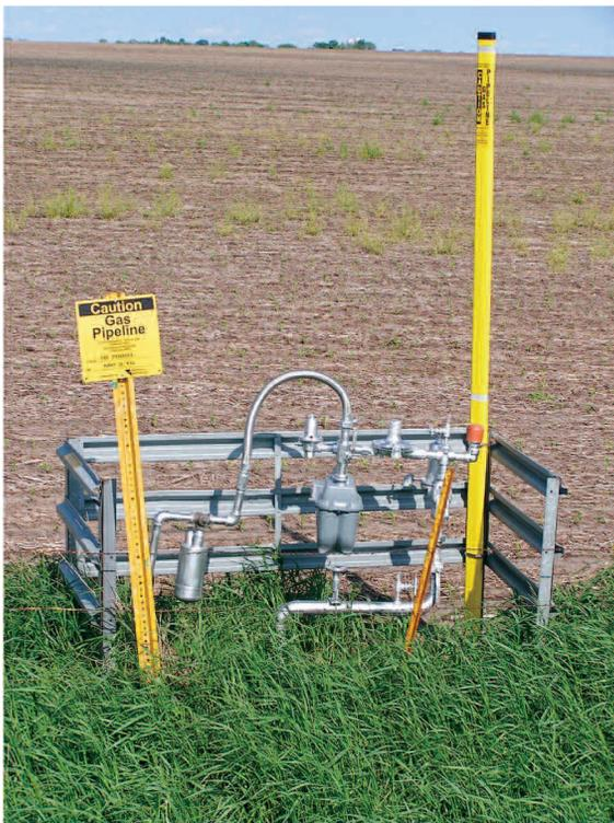
Our records indicate that you receive natural gas through a setting commonly referred to as a Farm Tap. These natural gas settings are made up of valves, pipes, regulators, relief valves and a meter. It may be located near your home or within the general vicinity. If the setting is in or near a cultivated field, a high visibility marker will make the setting easier to see. Call us to replace or install a marker.
